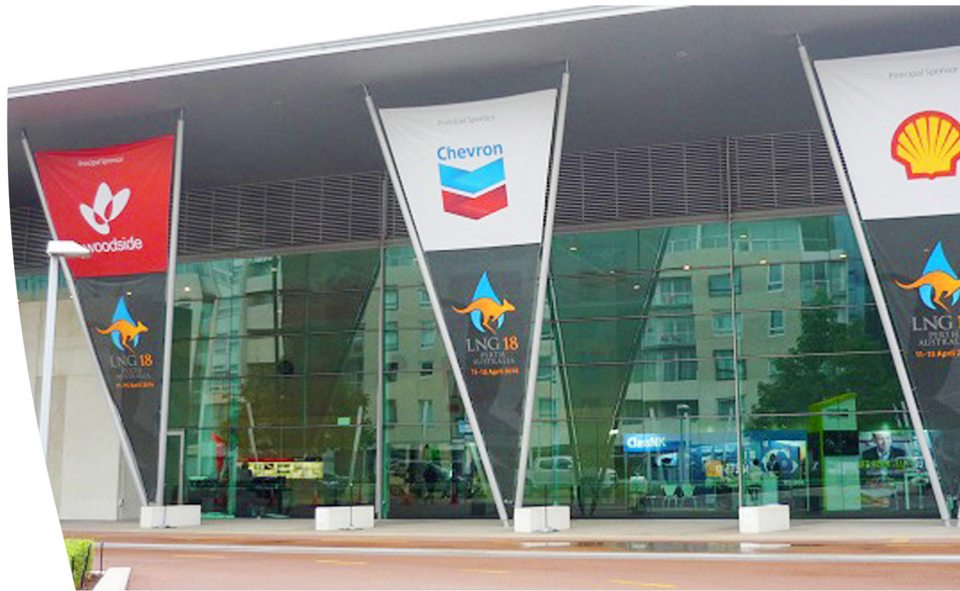
V-poles outside Level 1 Plaza
